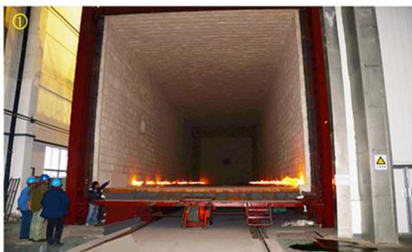
36m×7.4m×7.6m热处理炉 Heat Treatment Furnace(36m×7.4m×7.6m )
